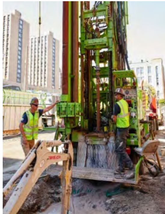
Pictured: Drilling of test wells; Courtesy of Dave Green Photography
